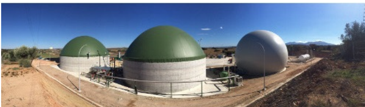
Figure 1: Campillos Biogas plant
